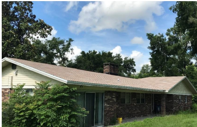
New roof funded by SHIP program.
