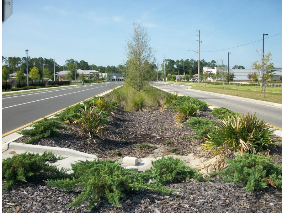
Bioretention median on NW 140th Street just north of Newberry Road
